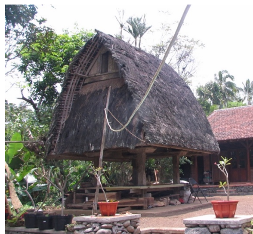
Figure 6. Granary/Jineng Buildings Source: Survey, 2019.
