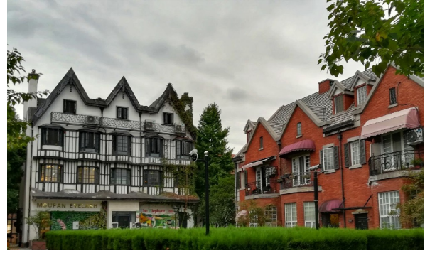
Figure 9: Different British-themed facades in Zone 2
