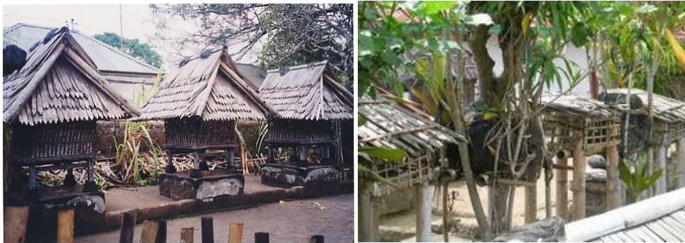
Figure 4: Buildings in Sacred Zone
