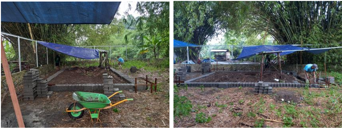
Figure 8: Foundation Construction
