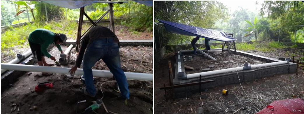
Figure 10: Tie foundation beams Process
