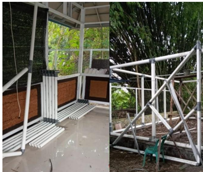
Figure 14: truss frames installations
