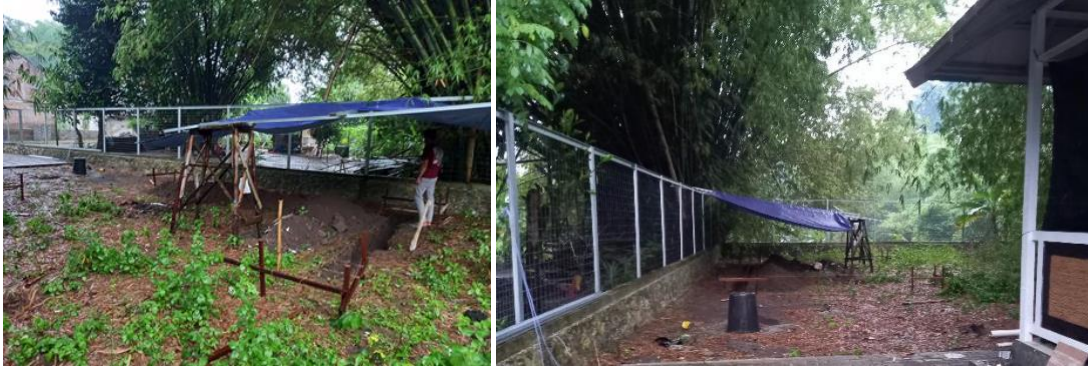
Figure 7: Excavation of Land
