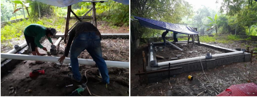
Figure 10: Tie foundation beams Process
